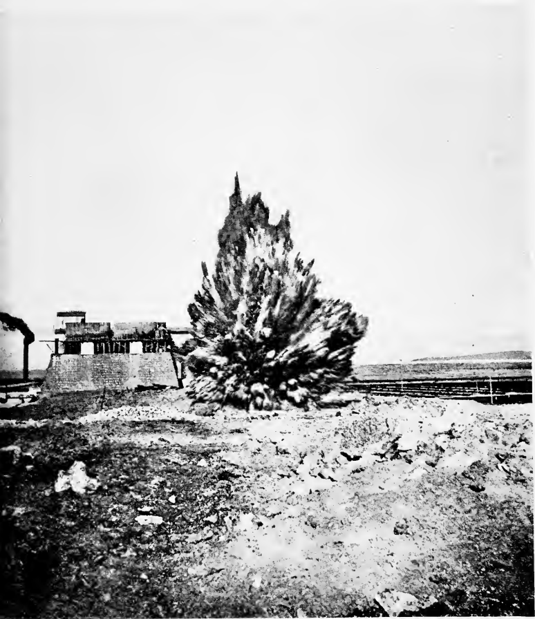
BLASTING A TEST HOLE, NITRATE FIELDS
